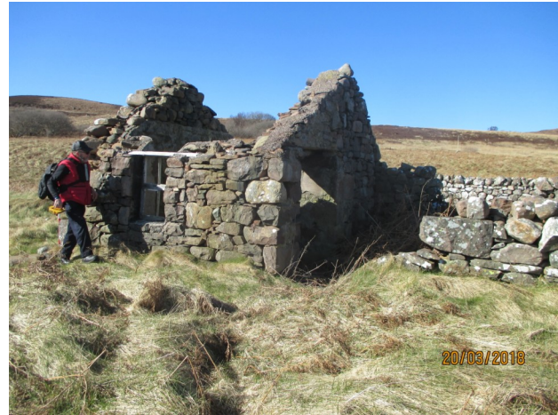
From the S. A building that has been altered
